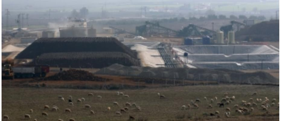
under one particular mode varying depending on the mineralogical characteristics of the laterite under test. The mineral extraction of the first trial heap has reached 78% nickel and 82% cobalt after some 15 months of irrigation, 72% for both metals was used in the bankable feasibility study.
